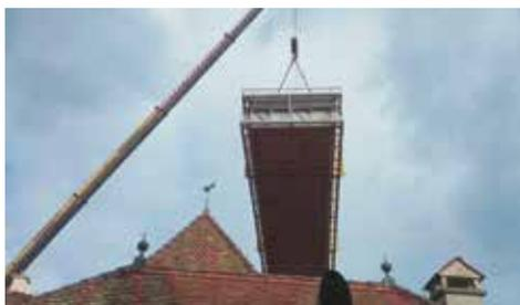
Facilities must have easy access (outside) to be able to install the crane that will help to unload the Spa or Pool and put it in place.
